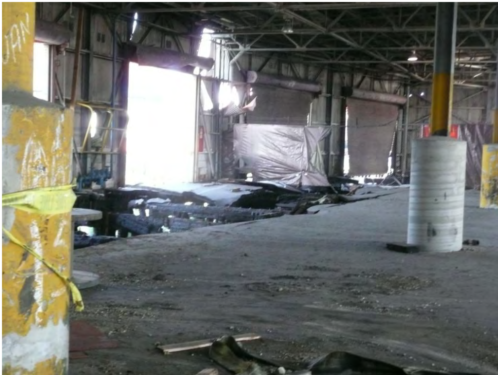
Figure 2-4d. Collapsing Floor and Fire-Damaged Metal Roll-up Doors
